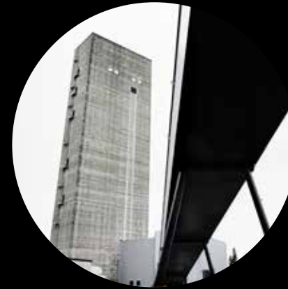
Headframe – ore hoist
