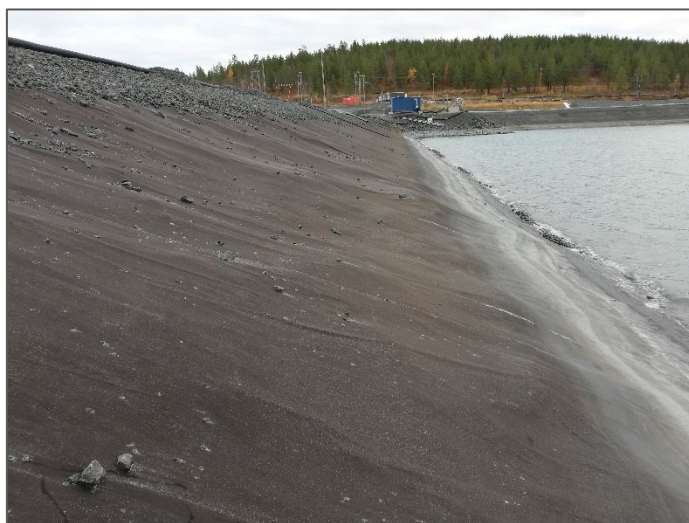
Kuva 18: Moreenin valumia kalvon alla altaan B pohjoisella padolla. / Downward movement of moraine (glacial till) under the membrane on the northern dam of TSF B.
