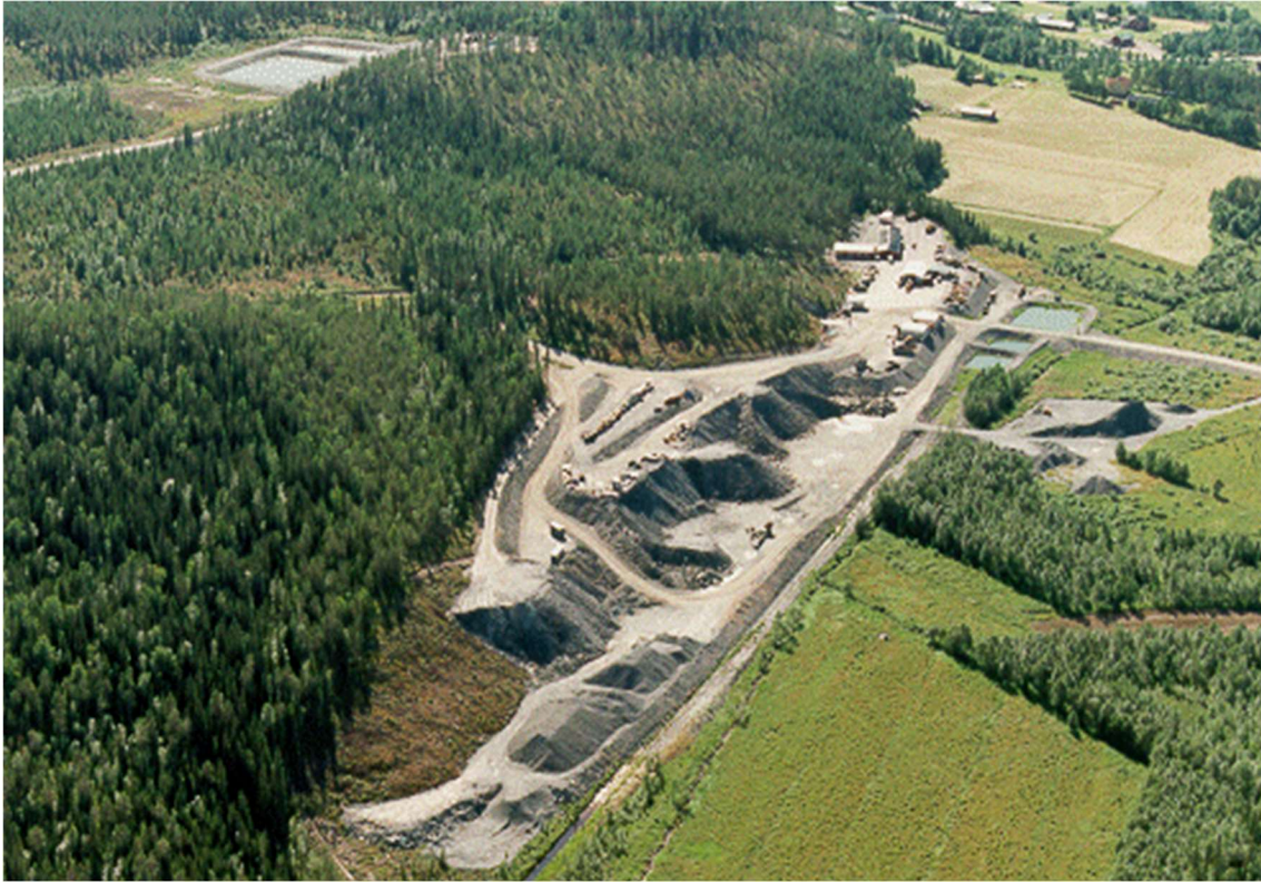
Front page: Picture showing Petiknäs mine site from 2007
