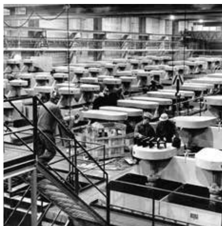
Assembly work in the flotation hall in Aitik, 1967.
