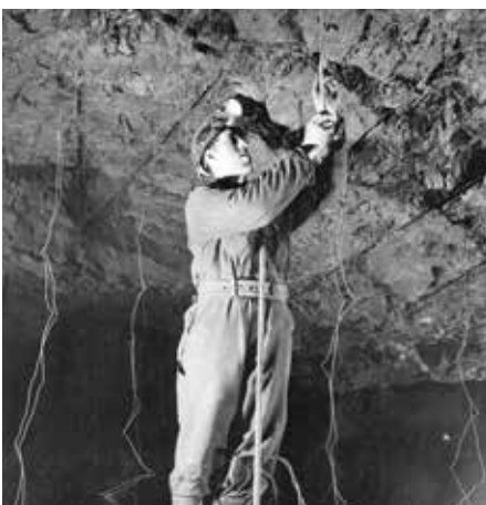
Priming a dynamite charge in Renström, 1955.
